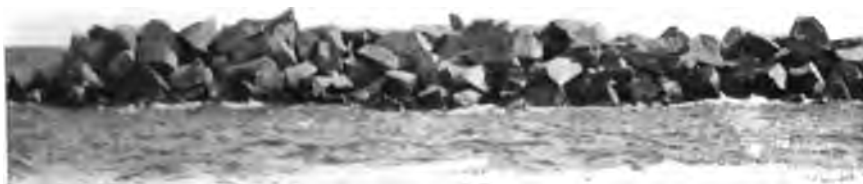
A SECTION OF THE BREAKWATER.
